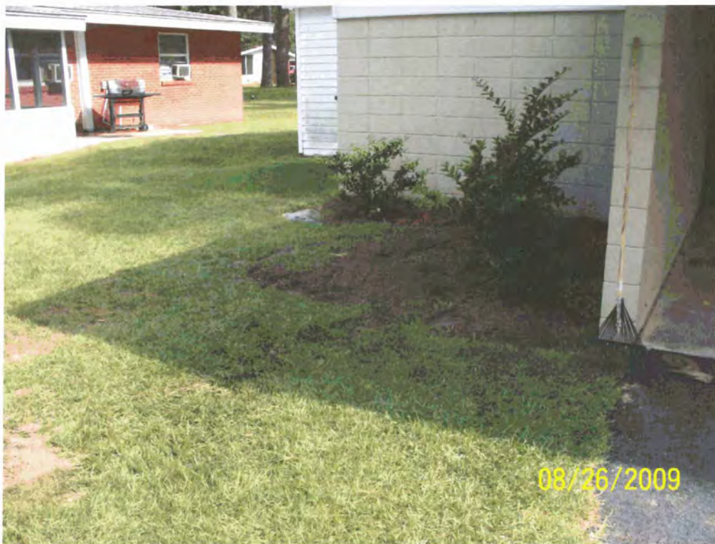
Picture 2: UST 1240Dove site after completion of work.
